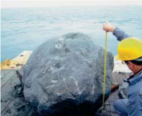
Figure 16. Boulders of considerable size were encountered.
